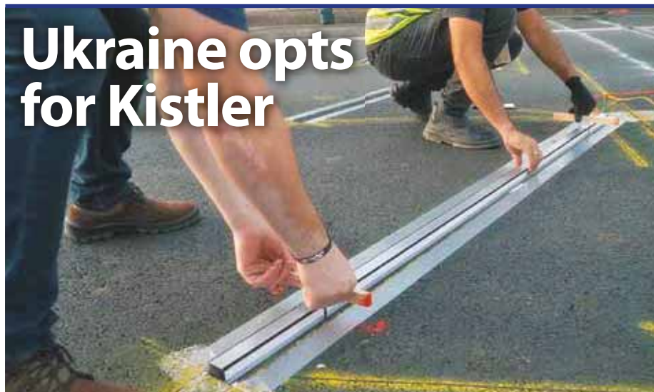
LEFT: Because of the slim shape of Kistler's Linesas quartz WIM sensors no massive cuts in the road are necessary for installation (image courtesy Kistler Group)
