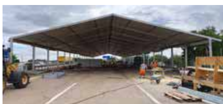
TOP & ABOVE: Kontent Structures installed an 18.5m-wide by 335m-long tent along the entire length of a bridge over the Rhine River in Karlsruhe, Germany, for work to continue regardless of weather (image courtesy Kontent Structures) BELOW: In the case of extremely cold weather, sandwich panels and air-filled double-layered roof covers can be used to provide insulation (image courtesy Kontent Structures)
