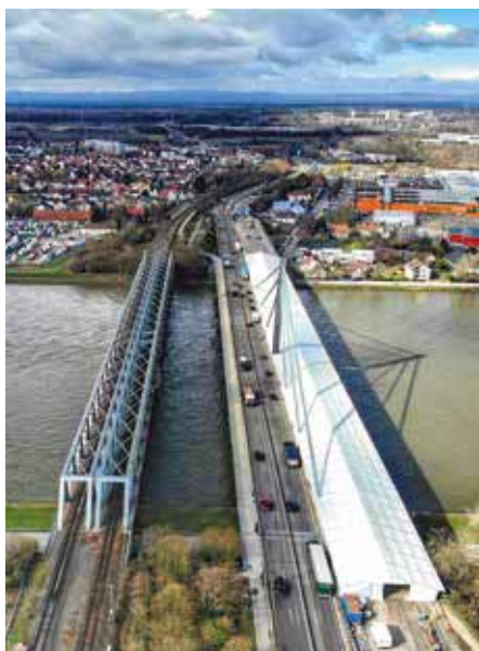
TOP & ABOVE: Kontent Structures installed an 18.5m-wide by 335m-long tent along the entire length of a bridge over the Rhine River in Karlsruhe, Germany, for work to continue regardless of weather (image courtesy Kontent Structures) BELOW: In the case of extremely cold weather, sandwich panels and air-filled double-layered roof covers can be used to provide insulation (image courtesy Kontent Structures)
