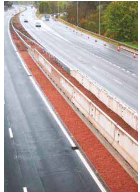
REBLOC RB140 and Maxibloc barriers were installed along Scotland's M8 motorway
